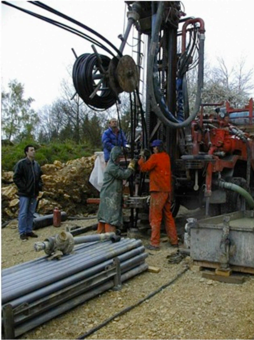
BHE drilling and installation
